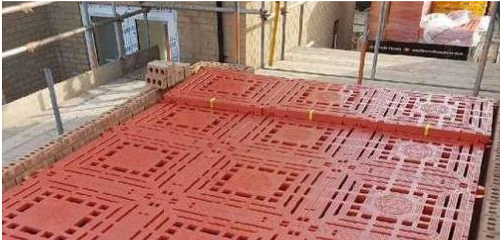
Figure 10 Macdeck 1x1 Panels with strapping
